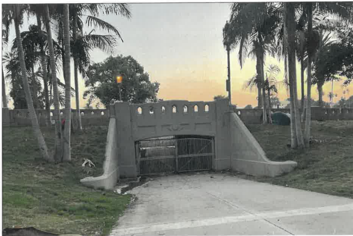
Figure 7. MacArthur Park gated pedestrian tunnel under Wilshire Blvd. 2023, Photo Courtesy of Office of Councilmember Eunisses Hernandez, City Council District 1, Photo by Louie Leiva
