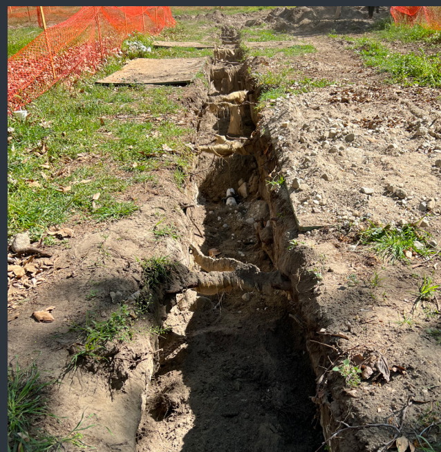
Tunneling under California sycamore roots at Arroyo Seco Ave 60 Park.
