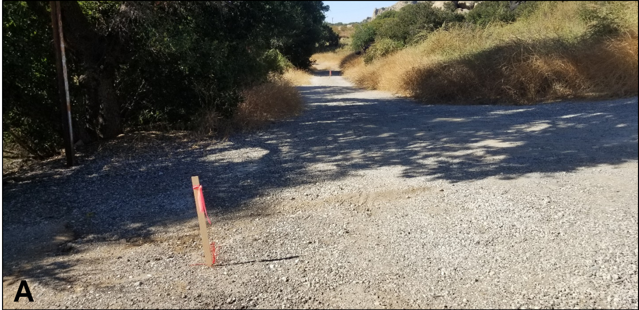
Photo A, facing south, showing survey markers for proposed trenching of the pipeline.
