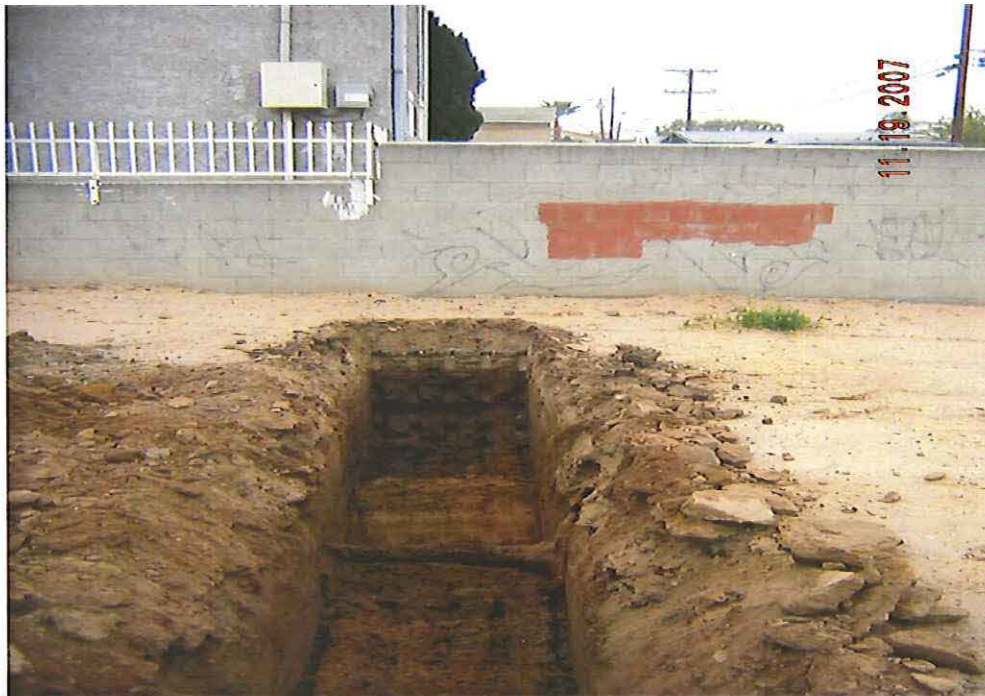
Looking south at a 2" pipeline that was discovered approximately 24" bgs.
