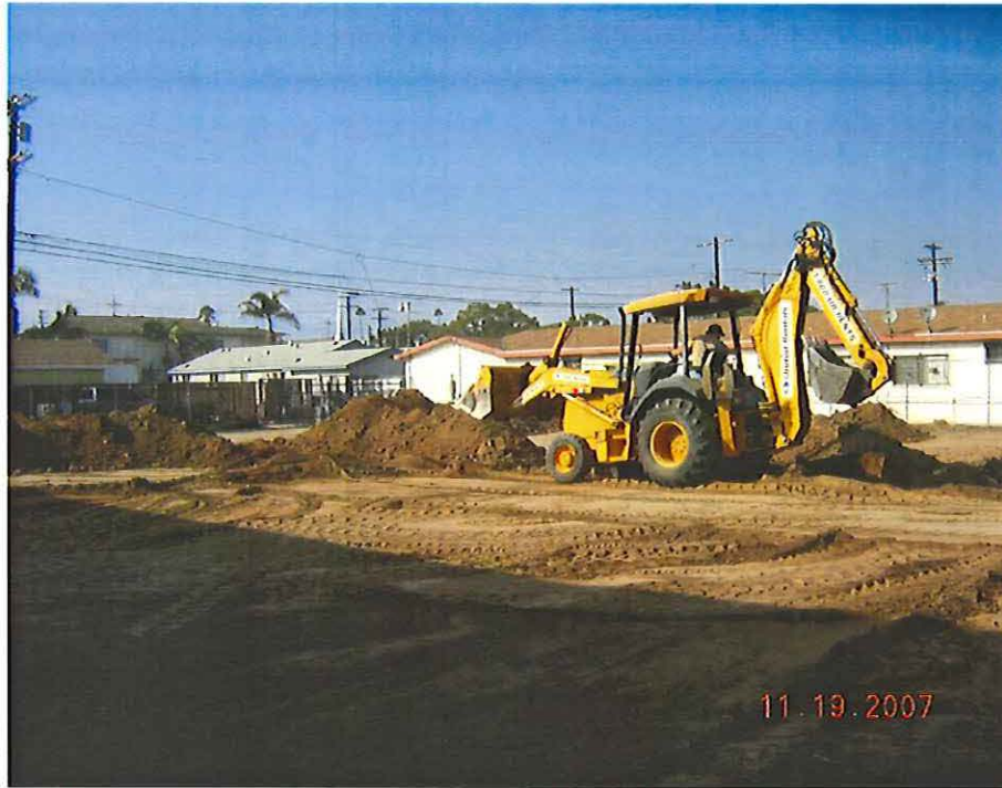
Looking northwest as the trenches were being backfilled and compacted.
