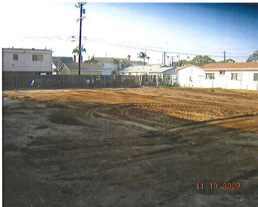
Looking northwest after completion of backfilling, grading, and compacting soil.
