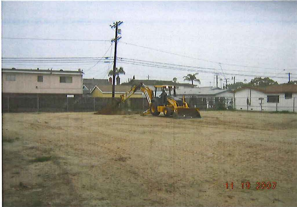
Looking west as trenching moves east.
