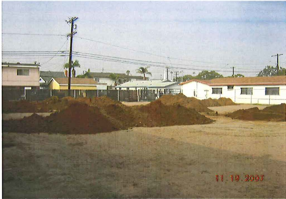
Looking west at trenching piles.
