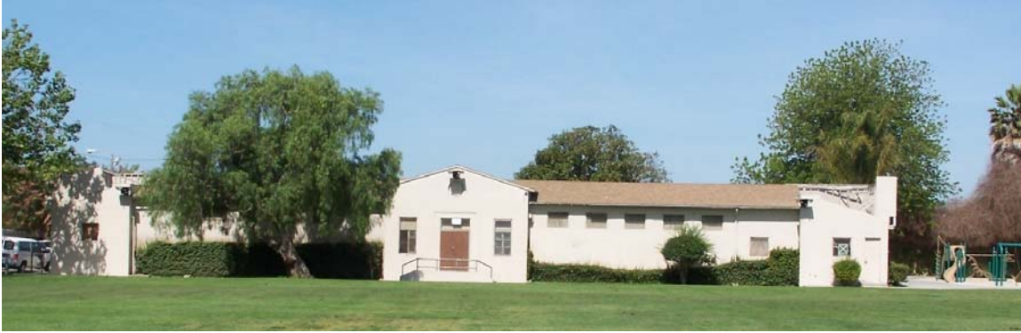
Figure 1: Bathhouse, east façade. 6 June 2007. Jones and Stokes.
