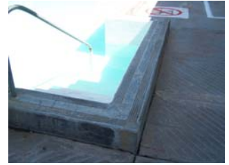
Figure 5: Pool, showing original etched coping and scored deck. 6 June 2007. Jones and Stokes.
