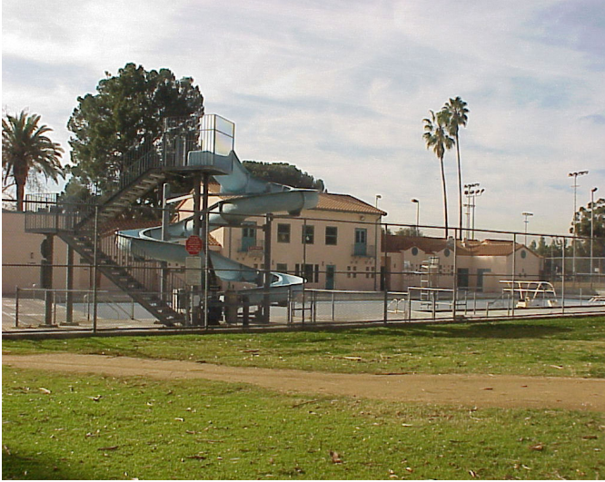
This older pool in Sun Valley, in fairly good condition, is testimony to the longevity in our pools with the experienced care and periodic refurbishment performed by Recreation and Parks Facility Repair staff.
