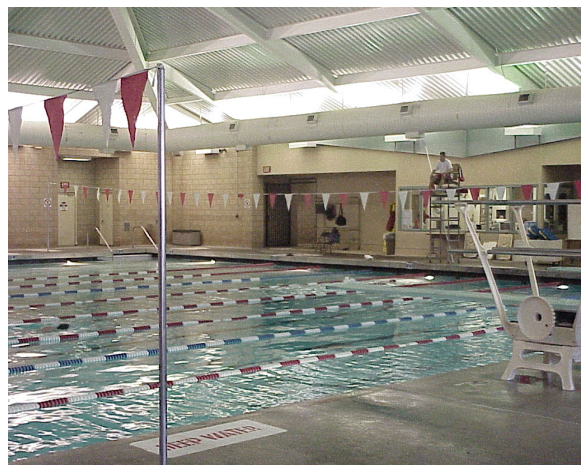
Cleveland is a newer pool, but the bathhouse, HVAC, and electrical room need major renovation.
