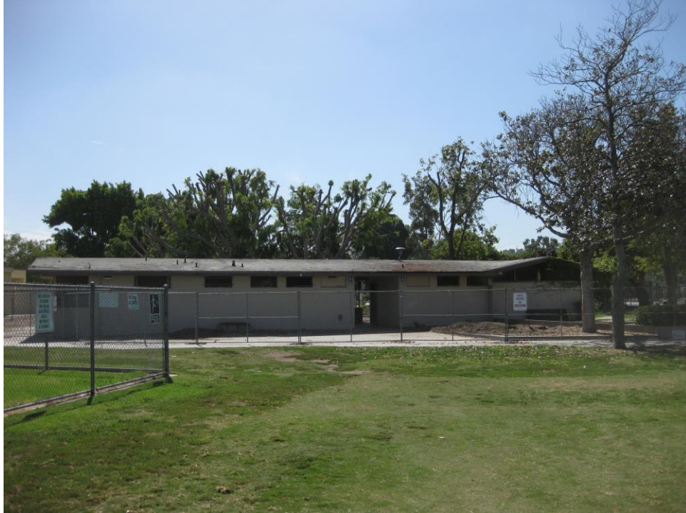
Plate 9. Restroom Facility, north side, view facing south
